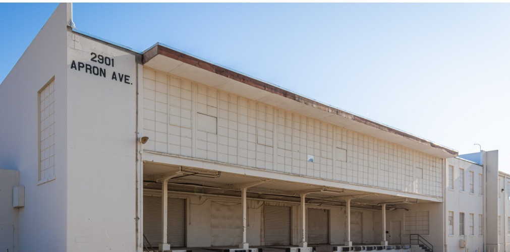
Ground-Level View: Dock-High Doors
