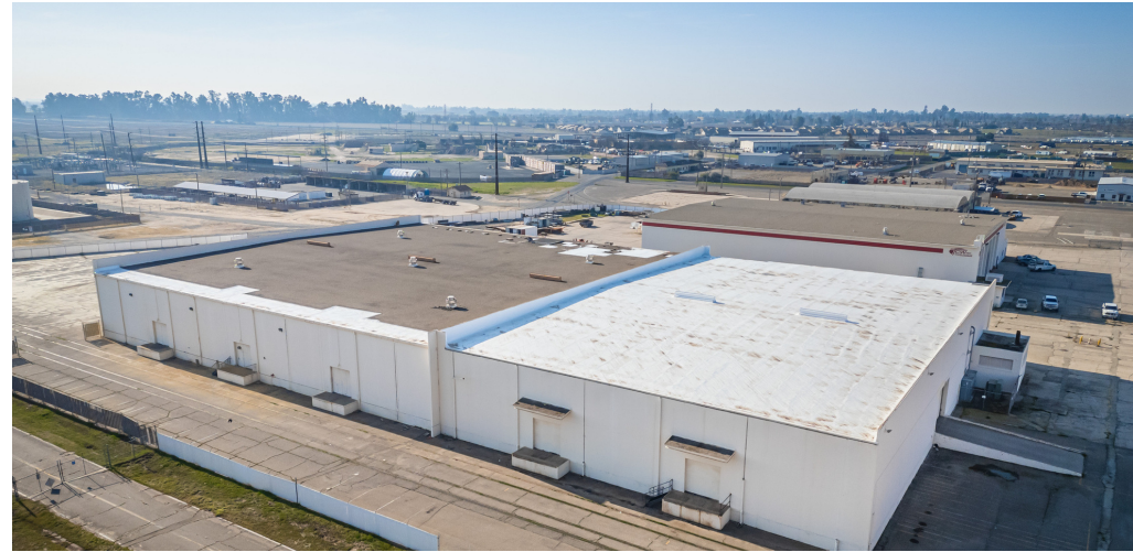
Aerial View: Rail Doors, On-Site Rail Spurs, and Recently Replaced Roof
