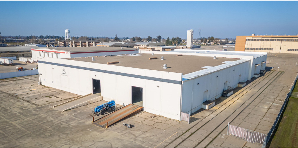
Aerial View: Grade-Level Ramp Doors and On-Site Rail Spurs
