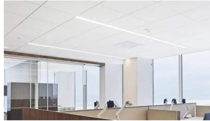
LINEAR LIGHTING IN ACT CEILING FOR OFFICE AREA: ARMSTRONG, 6' OR 8' O.C. LINEAR LIGHT FIXTURE
