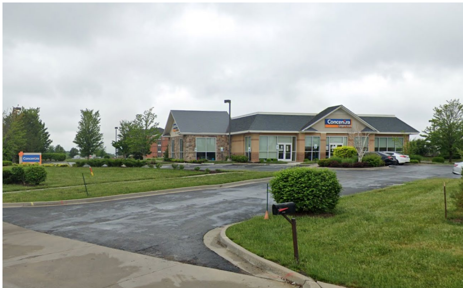
Subject property — 15430 S. Rogers Road, Olathe, KS. Stone & brick exterior with I-35 frontage.
