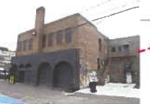
View looking toward SW building corner
