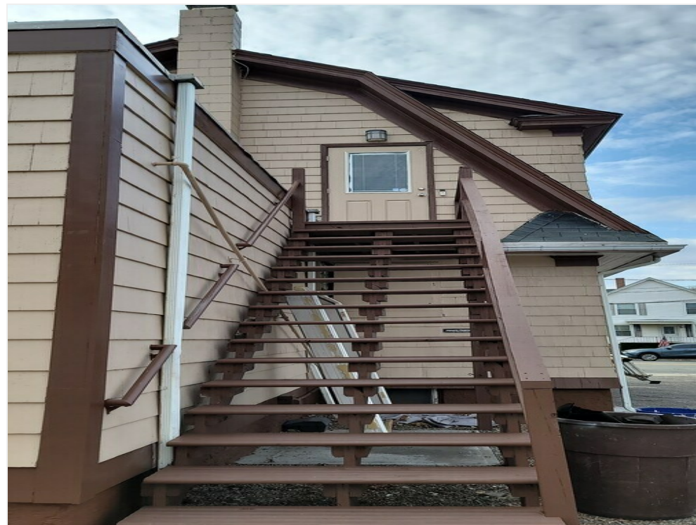
2nd Floor Rear Entrance
