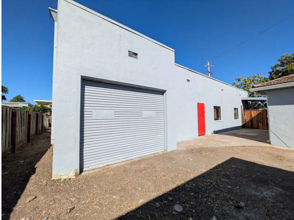
Interior Lot Warehouse
