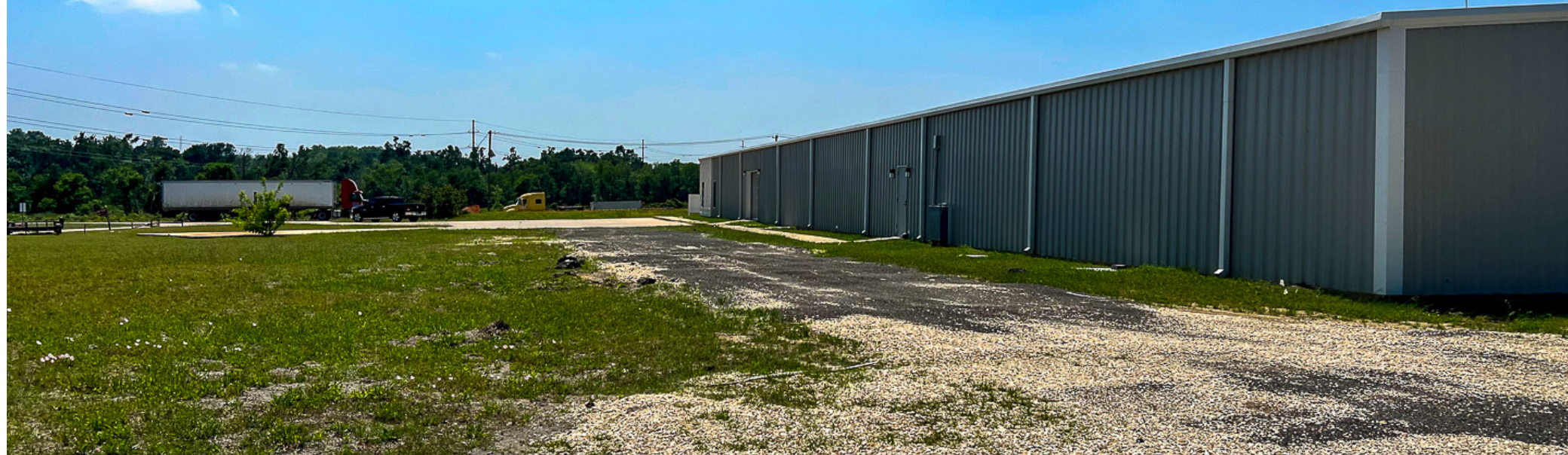
Back side of building, facing west
