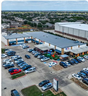
Shoppes at Westpark
