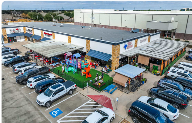
Shoppes at Westpark
