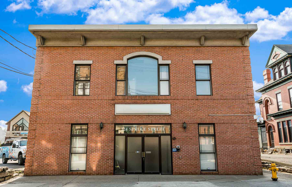
Front View of the Building.
