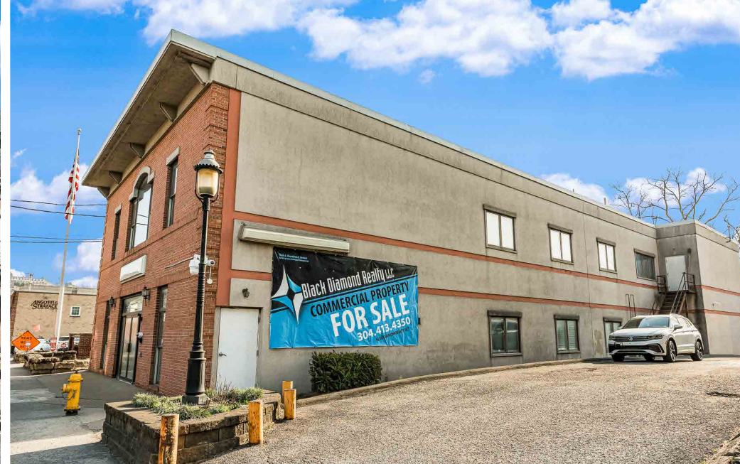
Side View of the Building.
