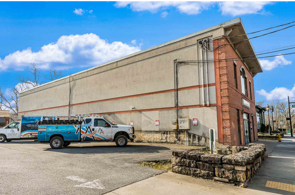
Side View of the Building.
