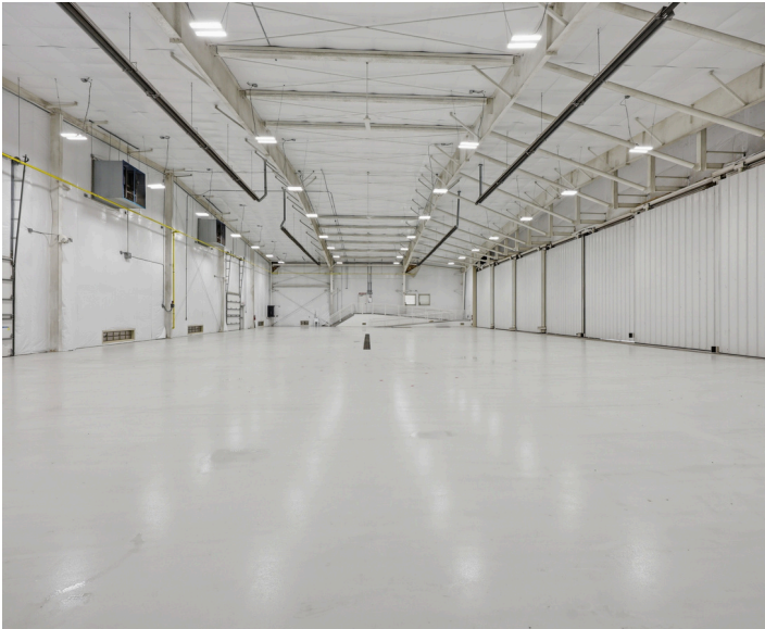
MAIN BAY · CLEAR-SPAN INTERIOR
