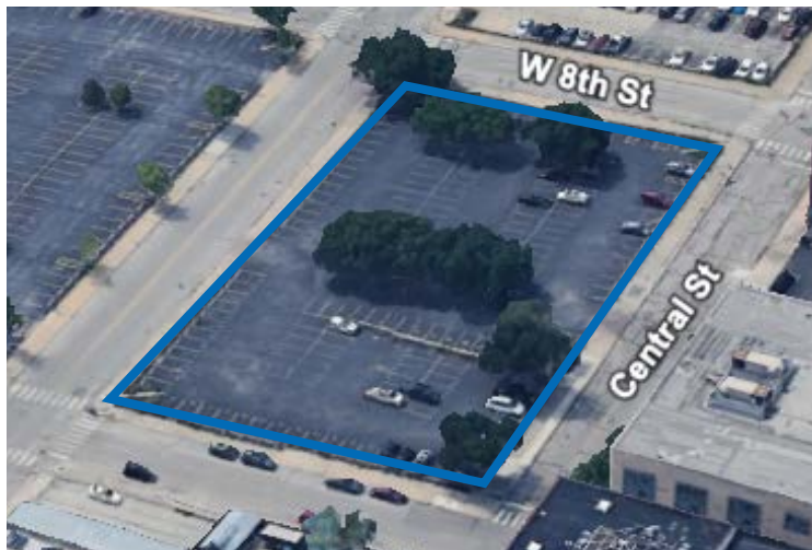
700 WYANDOTTE STREET AND 701 CENTRAL STREET
