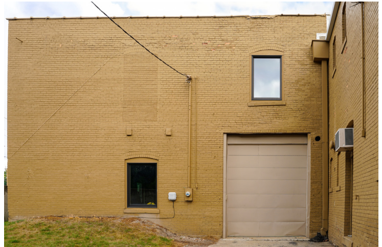
Rear overhead door
