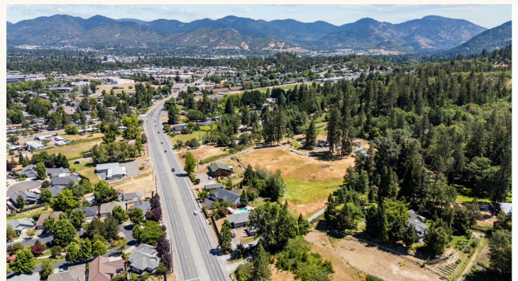
Corridor and valley context — south Grants Pass rooftops beyond.
