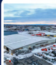
206 PLAINVIEW INDUSTRIAL 80,000 SF WAREHOUSE
