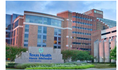
Texas Health Harris Methodist Hospital
