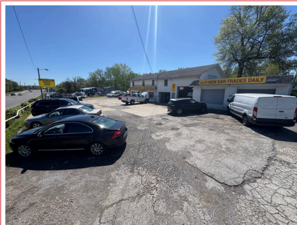
Front lot + 3,500 SF building + garage.
