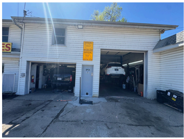
The shop. Five D.I. doors total.
