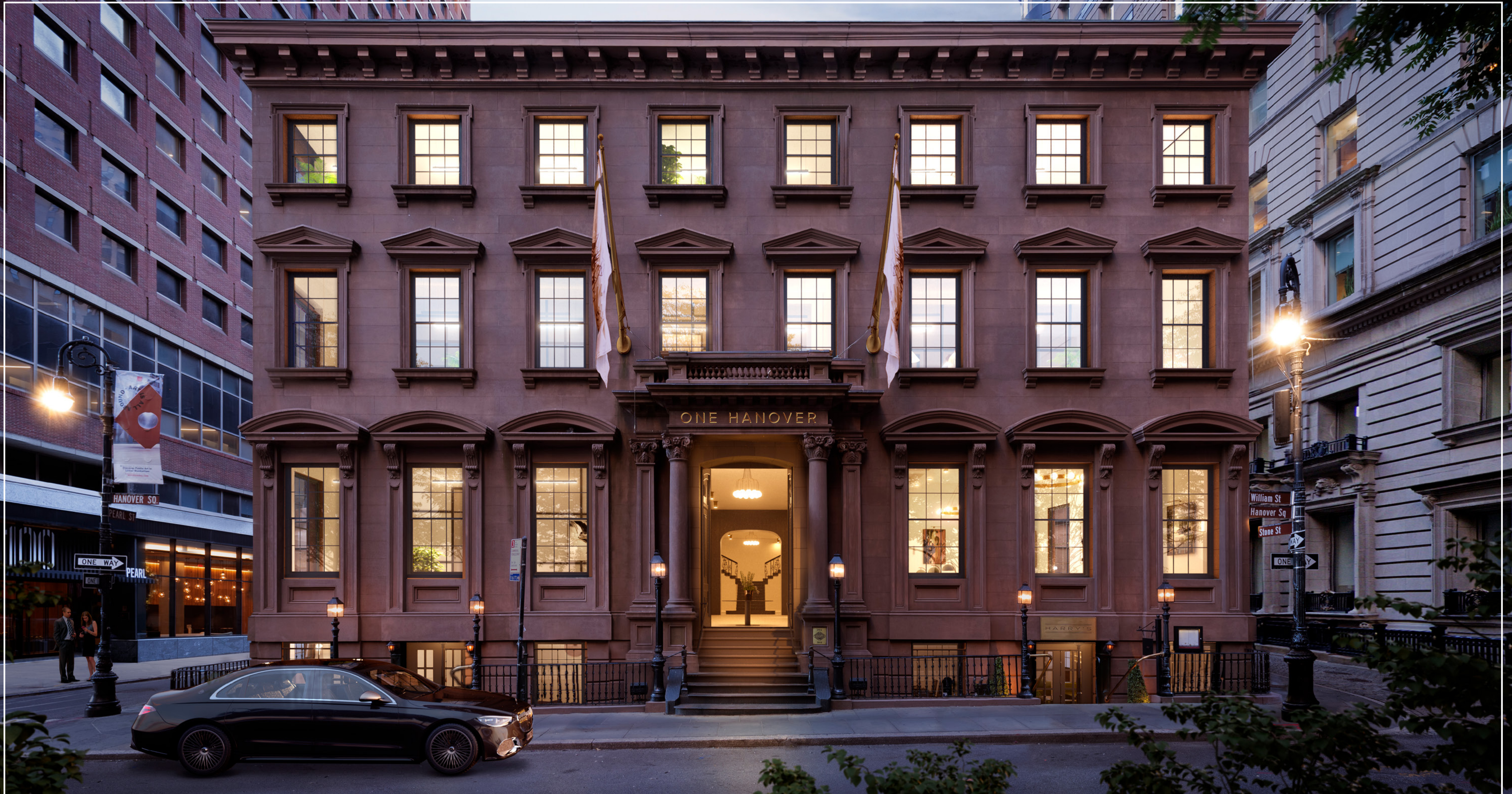
LANDMARK 3-STORY BUILDING
