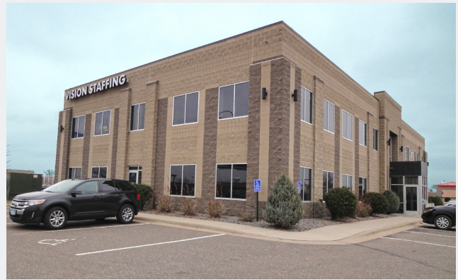
Building Signage Available Along I-94
