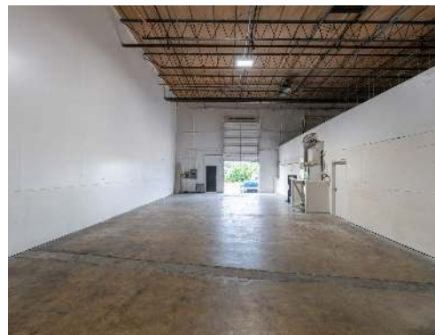
Existing dock door — knock-out panel for additional door
