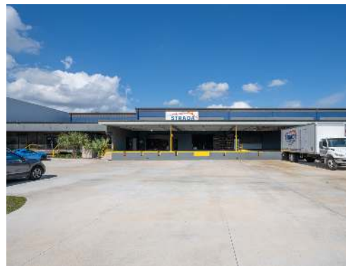
Covered dock-high loading canopy
