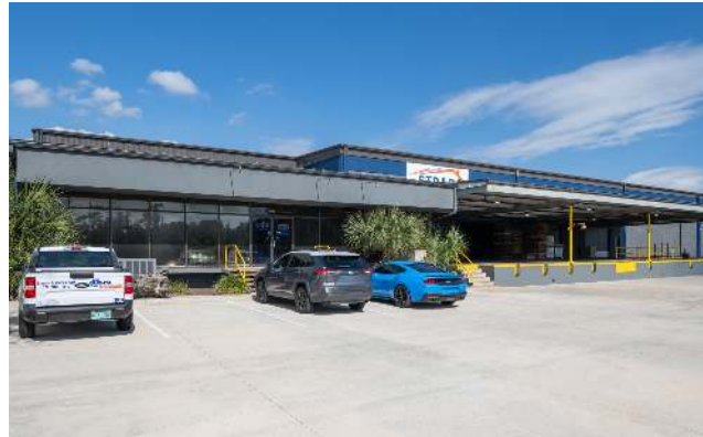
Building Frontage & Storefront
