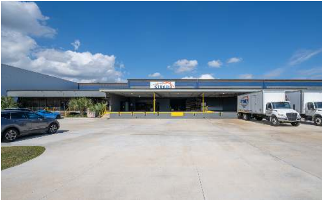
Covered Dock-High Loading Canopy
