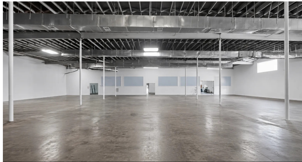
Fully Conditioned – 17' Height – 15' x 32' Column Spacing
