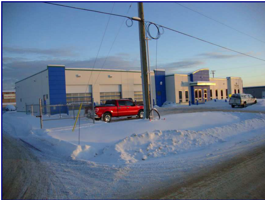
FRONT VIEW OF SUBJECT BUILDING • LOOKING SOUTHEAST
