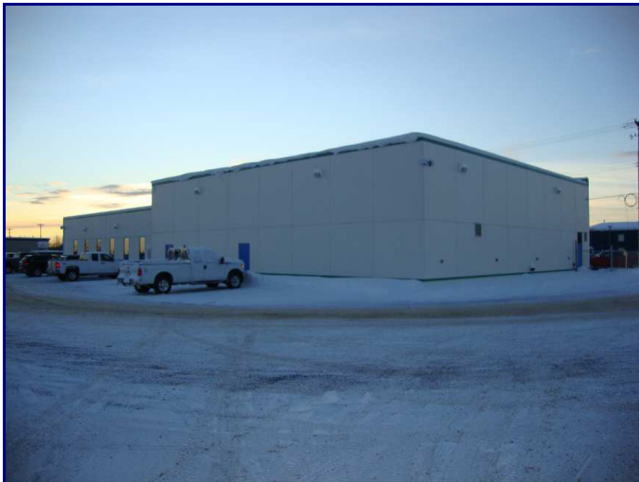
REAR VIEW OF SUBJECT BUILDING • LOOKING NORTHWEST
