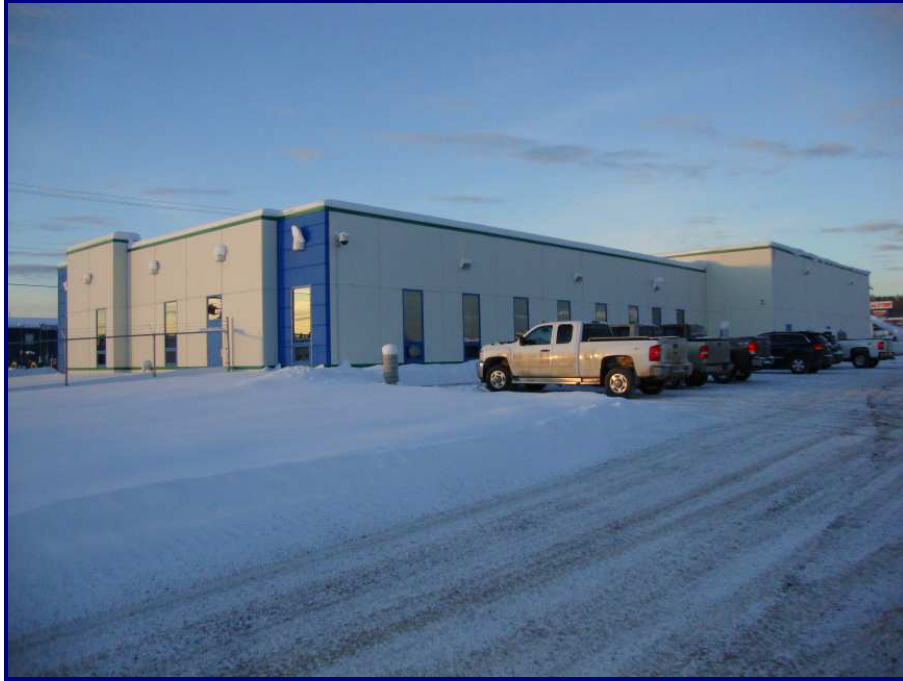
REAR VIEW OF SUBJECT BUILDING • LOOKING NORTHEAST
