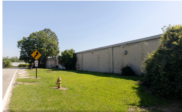
Side elevation and street frontage
