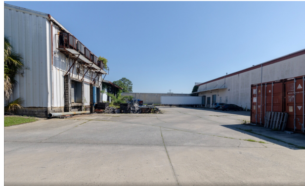
Interior yard between buildings with dock access
