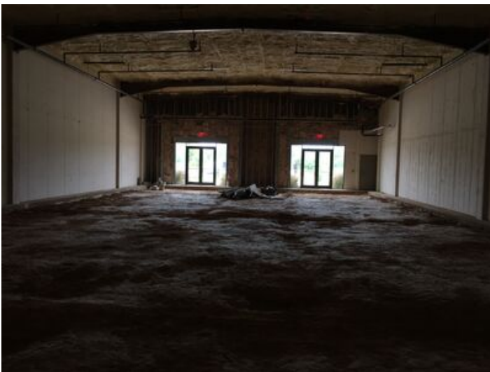
Interior Bays B&C 2400 sq
