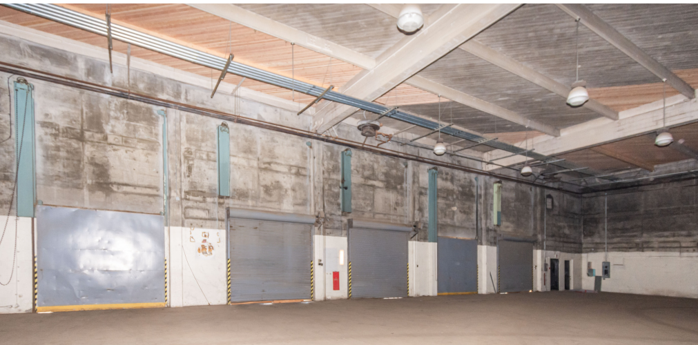
Unit B: Five (5) Dock-High Doors and Recently Replaced Roof
