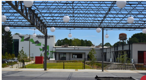
Exposed trusses and open-air entry to create view corridor. Flanked by outdoor restaurant spaces and seating, featuring local art and landscaping
