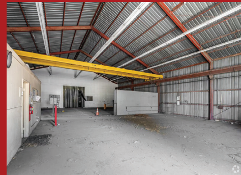
(65' x 175') INSIDE FRONT BUILDING
