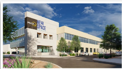
New Space Nexus (Under Construction)
