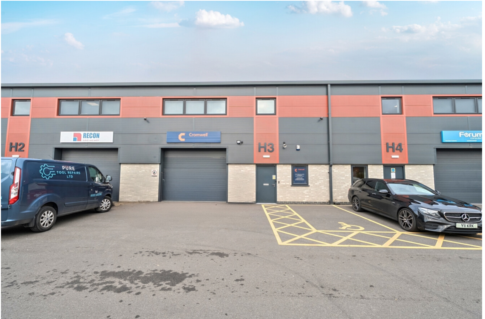
H3 Hybrid Unit Leafbridge, Station Road, North Hykeham, Lincoln, Lincolnshire, LN6 3QX
