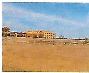
View of Site; New Apartments Immediately South
