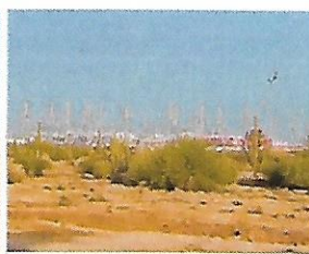
TSMC Cranes / Construction
