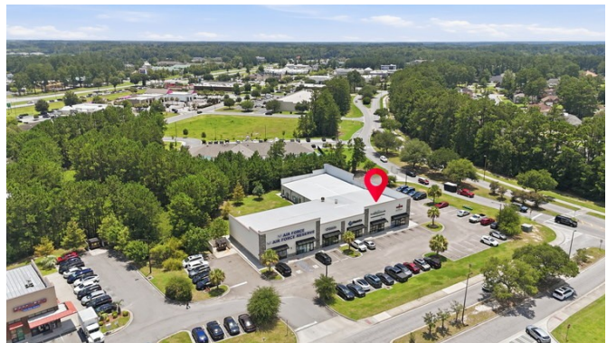
Hard-corner position with access from two roads
