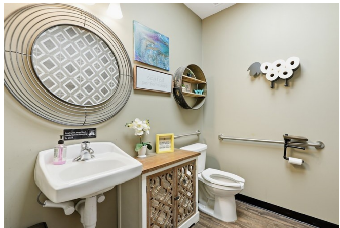
One of two restrooms — fixtures and ADA grab bars in place
