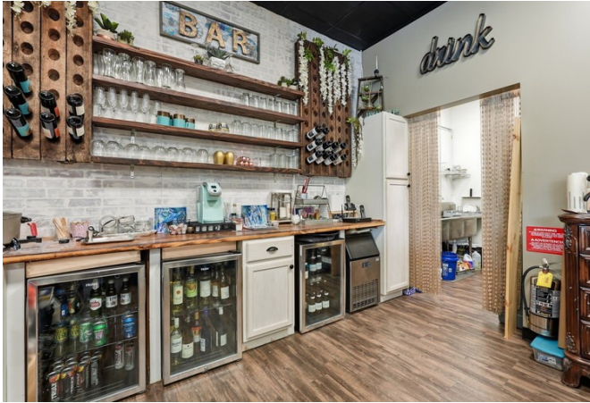
Bar area — water, waste and electrical connections in place
