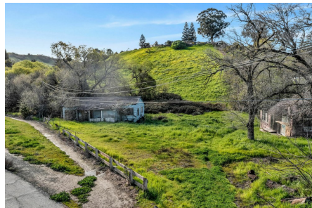
Ground Level — Existing Structures & Access Road
