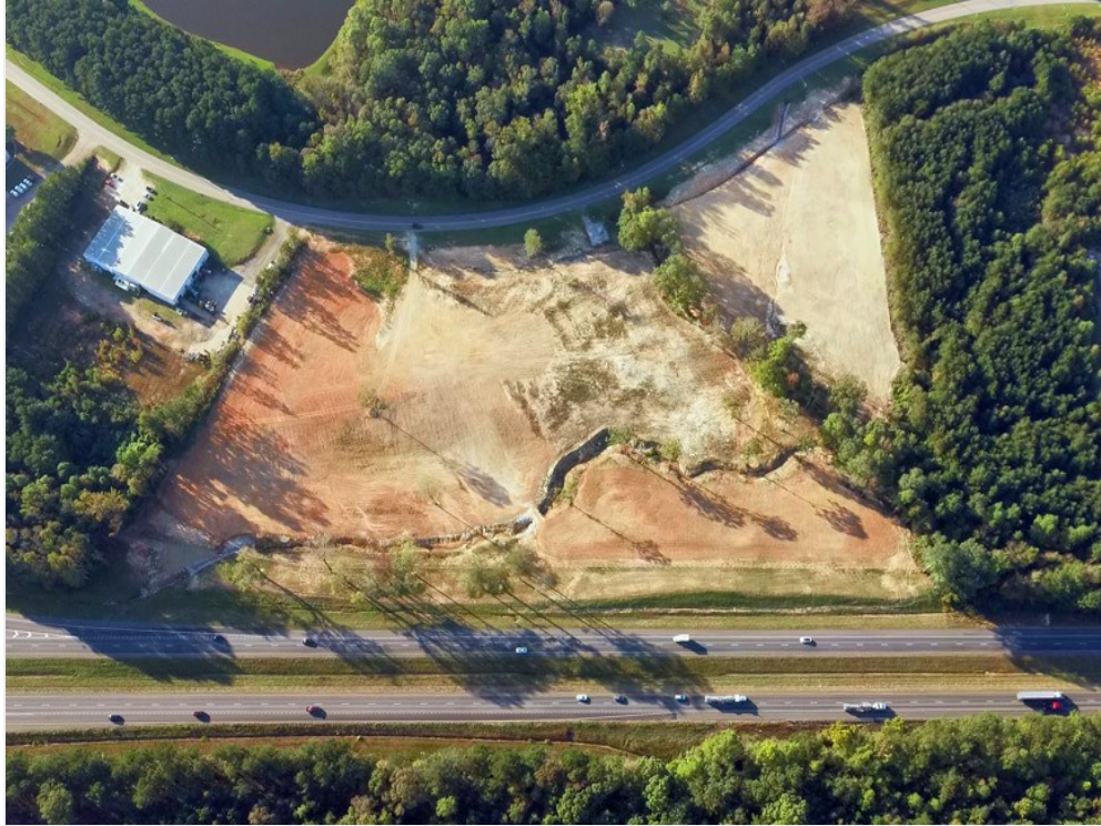
Building Exit 77 - Lanett
