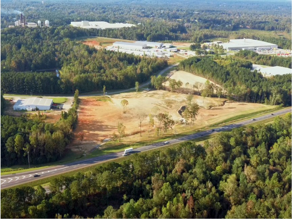
Building Exit 77 - Lanett
