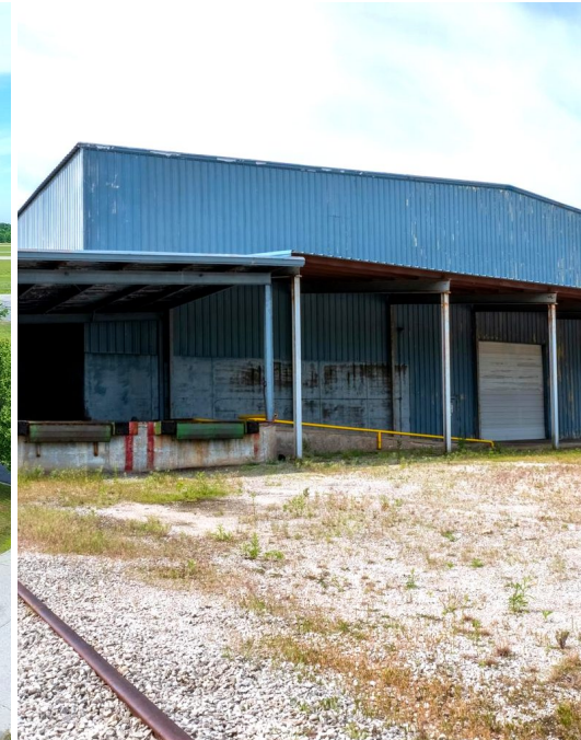
BNSF RAIL SIDING + DOCK
