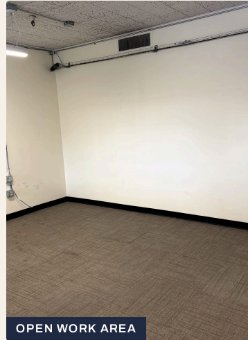
OPEN WORK AREA
