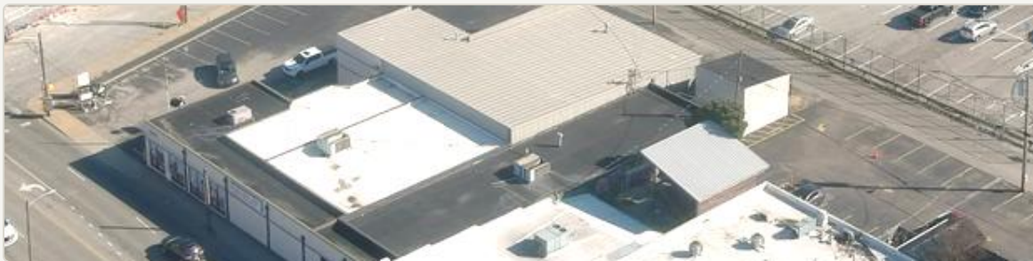
THE SUBJECT BUILDING · CHURCH STREET &amp; 15TH AVENUE NORTH
