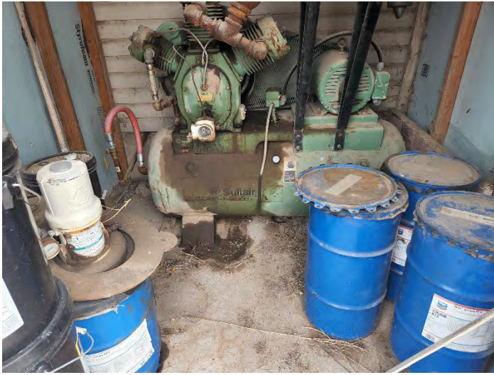
9. Compressor (minor staining no conduits to the subsurface)
