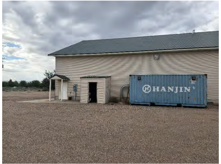
6. South side of the building
