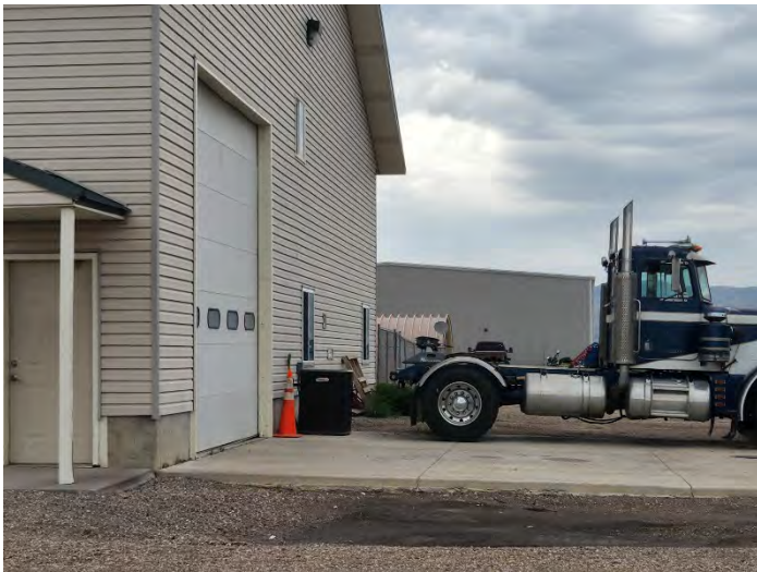
3. Delivery bay on the west side
