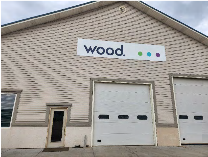
1. Overall view of the subject property
