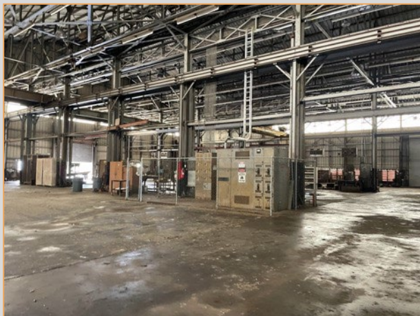
Maintenance shop interior
