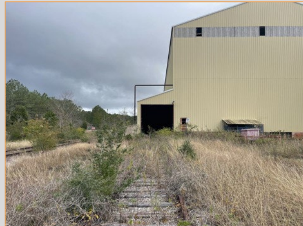
Rail access to main plant
