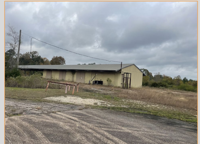
Vehicle Storage Building (F)
