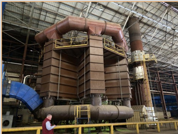
Main Plant Interior
