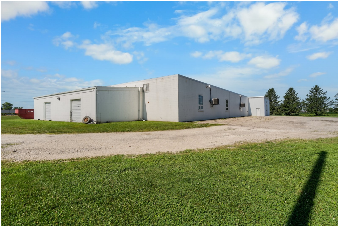
Warehouse elevation — grade-level overhead doors and truck-friendly yard access
