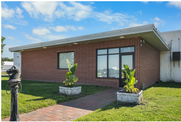
Brick office entrance & reception
