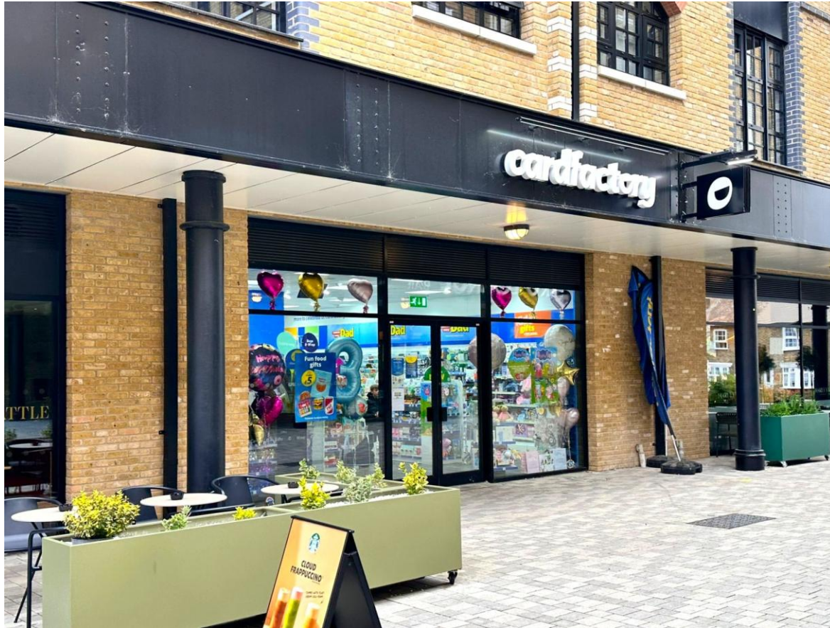
Unit 1A – Card Factory
