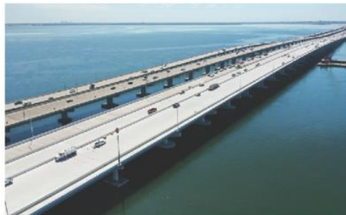
HOWARD FRANKLAND BRIDGE I-275
