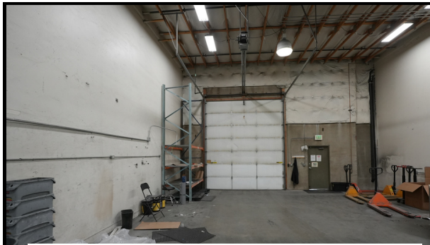
7 ground level doors (12'x14')
