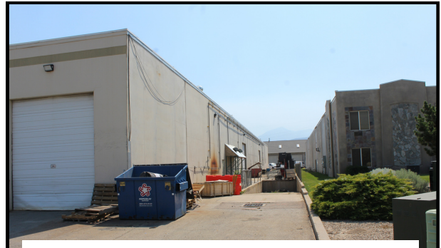
Shared loading dock
