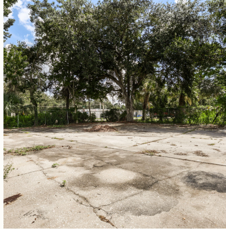
FENCED LAYDOWN YARD
