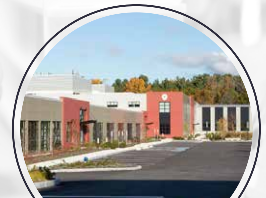
33 NEW YORK AVENUE, 1 & 5 MOUNTAIN ROAD FRAMINGHAM | 263,000 SF
