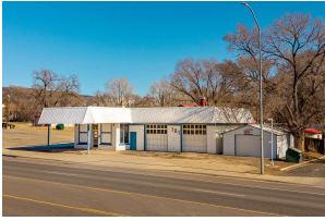
Front Of Structure
