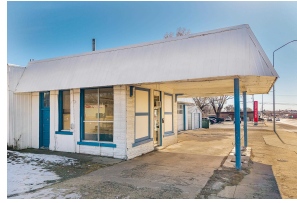
Front Of Structure
