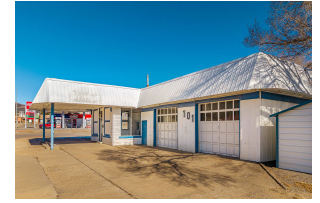
Front Of Structure
