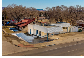
Front Of Structure
