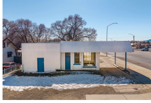
Front Of Structure
