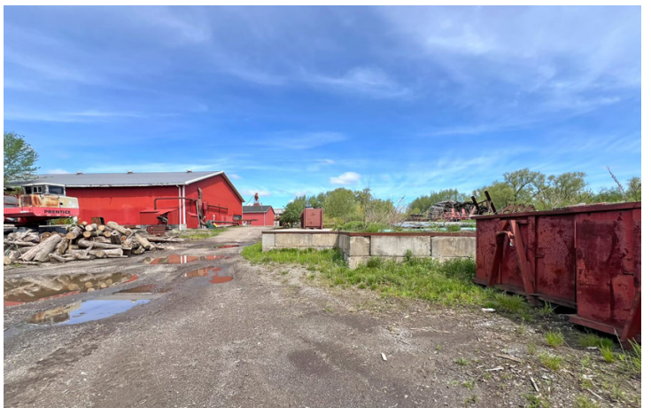
Loading Dock Platform
