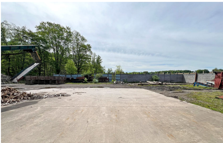
Partially Fenced Storage Yard
