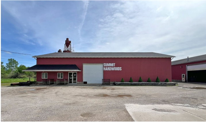
Bldg. 1: 4,200± SF Showroom/Warehouse With 16' Clear Ceilings, 3 Overhead Doors: (2) 12'x12' & (1) 18'W x 12'H & Reznor Gas Heat
