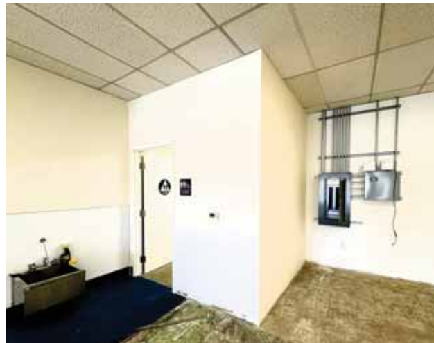
2842-#25 Story Road - Interior
