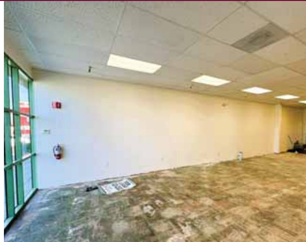
2842-#25 Story Road - Interior
