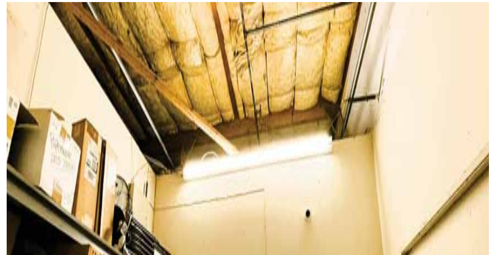
2842-#40 Story Road - Interior (Storage/Warehouse Area - Open Beam Ceiling)
