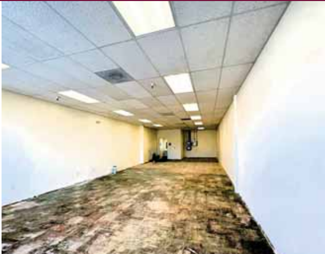
2842-#25 Story Road - Interior
