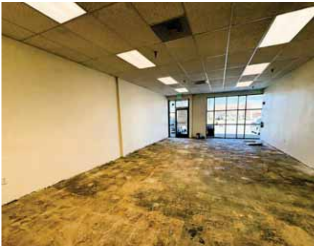
2842-#25 Story Road - Interior
