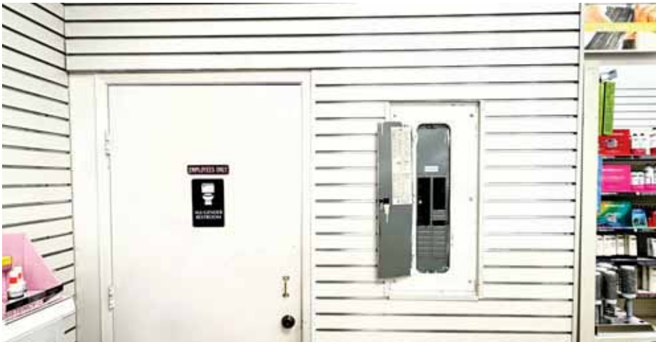
2842-#40 Story Road - Interior
