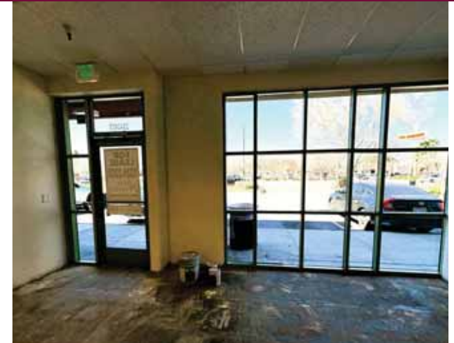
2842-#25 Story Road - Interior
