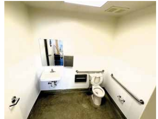
2842-#25 Story Road - Interior
