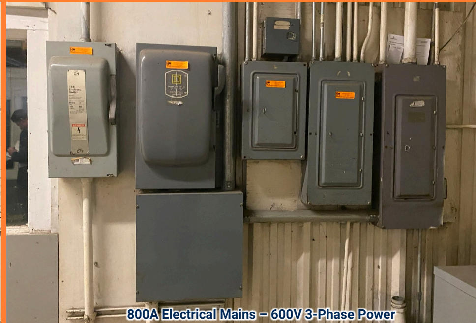
800A Electrical Mains - 600V 3-Phase Power
