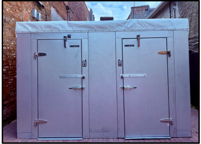
Exterior: 12x12 Walk-in Refrigeration & Freezer
