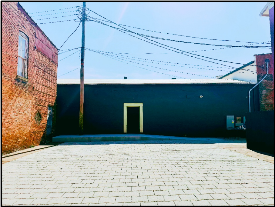
Exterior: Renovated 6 th Street Patio
