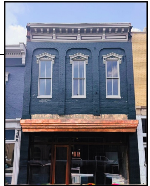
Exterior: Main Street Façade
