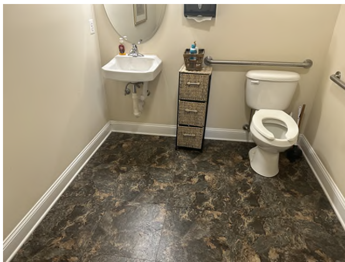
116 Interior (Lower Level)
