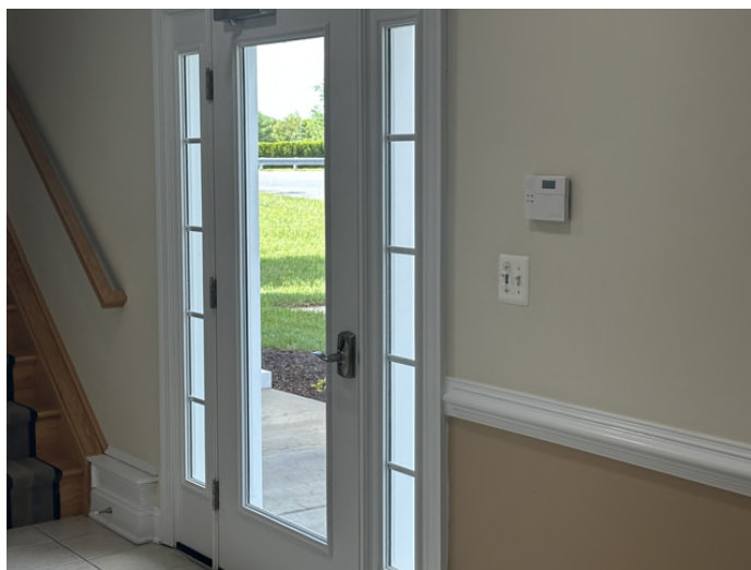
123 Interior (Lower Level)
