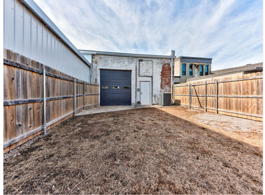
Back of Building
